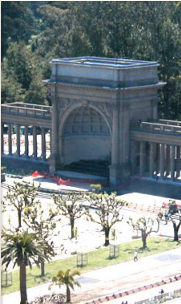
The Bandstand at Golden Gate Park
